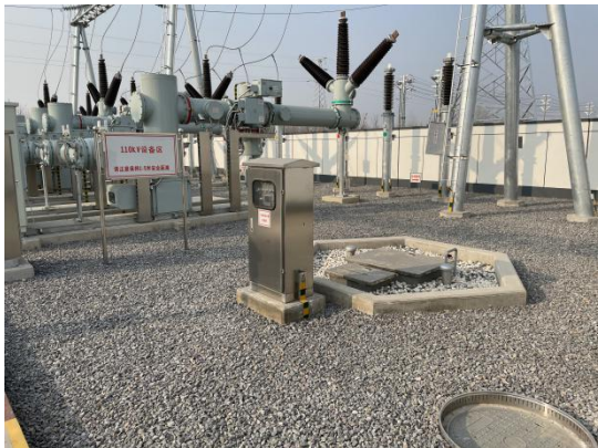
4-1 (b) 变电站区碎石铺垫
