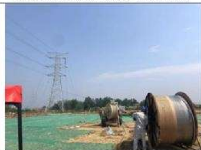
牵张场区编织布铺垫及钢板铺设 (2022.6.6)
