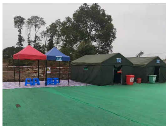
牵张及跨越场区防尘网苫盖
