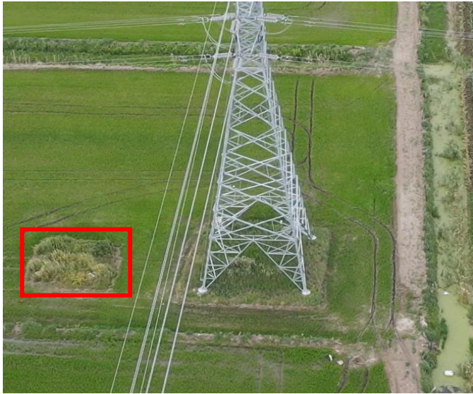
拆除塔基区撒播草籽 (2025.7)
